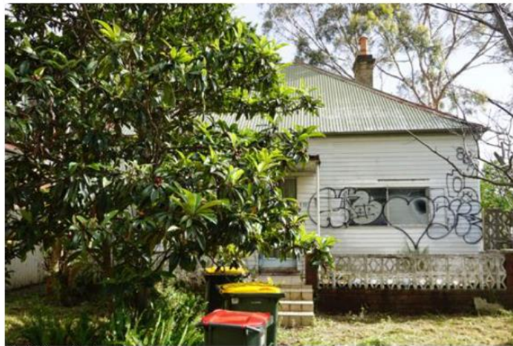
Fig.8 Street facing façade
