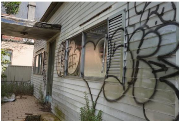
Fig.30 Street facing facade
