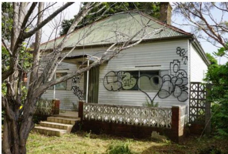
Fig.36 Street facing facade
